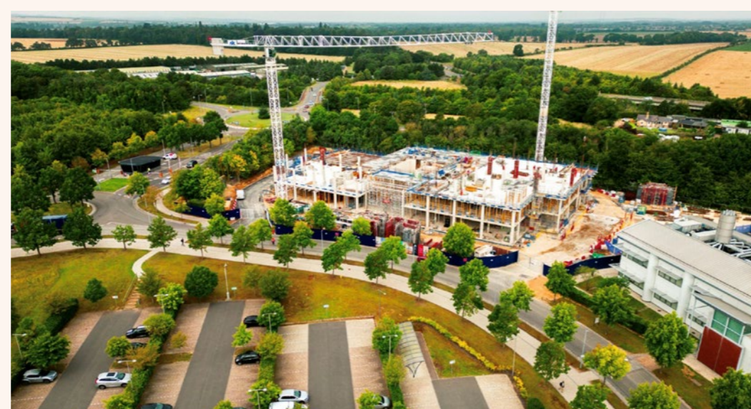
View of Site 1 construction underway
